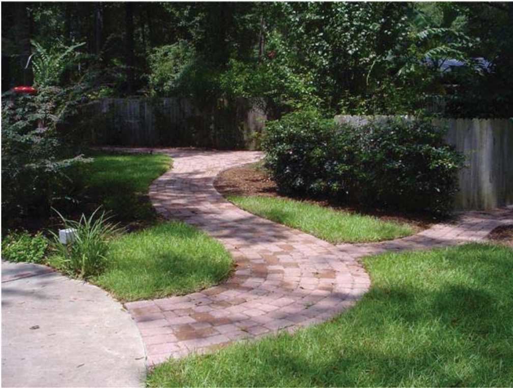
Figure 26. Permeable walks, such as this paver brick path installed on compacted base material, will allow rainwater to filter through or around the paved surface. These pathways can also make previously unreachable areas accessible to wheelchairs or strollers. Photo by Pat Drackett. Landscape contractor: GroundScape Inc., Biloxi.
